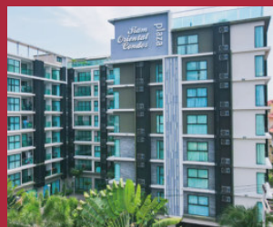
Plaza 190 units Completed 2018
